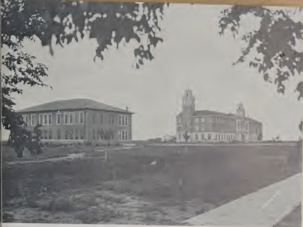
28. Home Economics Building and Administration Building on the Right.
